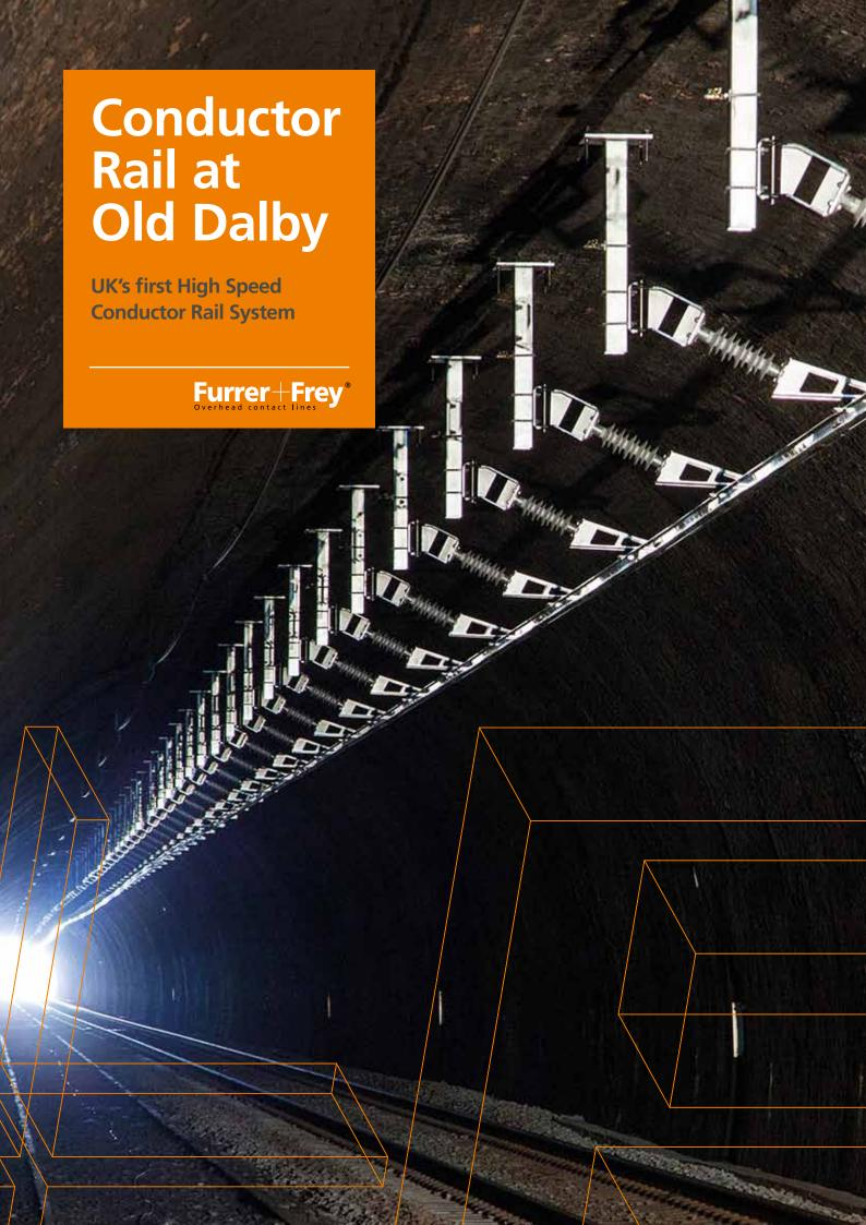
Stanton Tunnel on Old Dalby Test Track has been upgraded with Furrer+Frey Rigid Overhead Conductor Rail System (ROCS), making it UK's first for High Speeds (up to 140mph).
